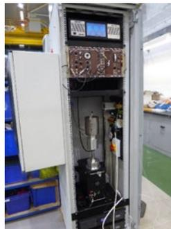
Gaseous Activity Monitoring (GAM) system at Hartlepool power station
